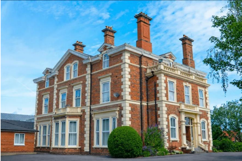
Nazareth House Birkenhead, main convent building
